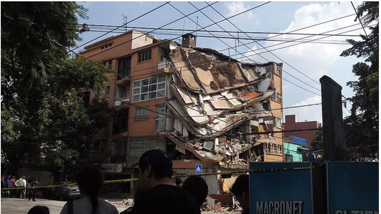
Building damaged by the 2017 Puebla earthquake.
